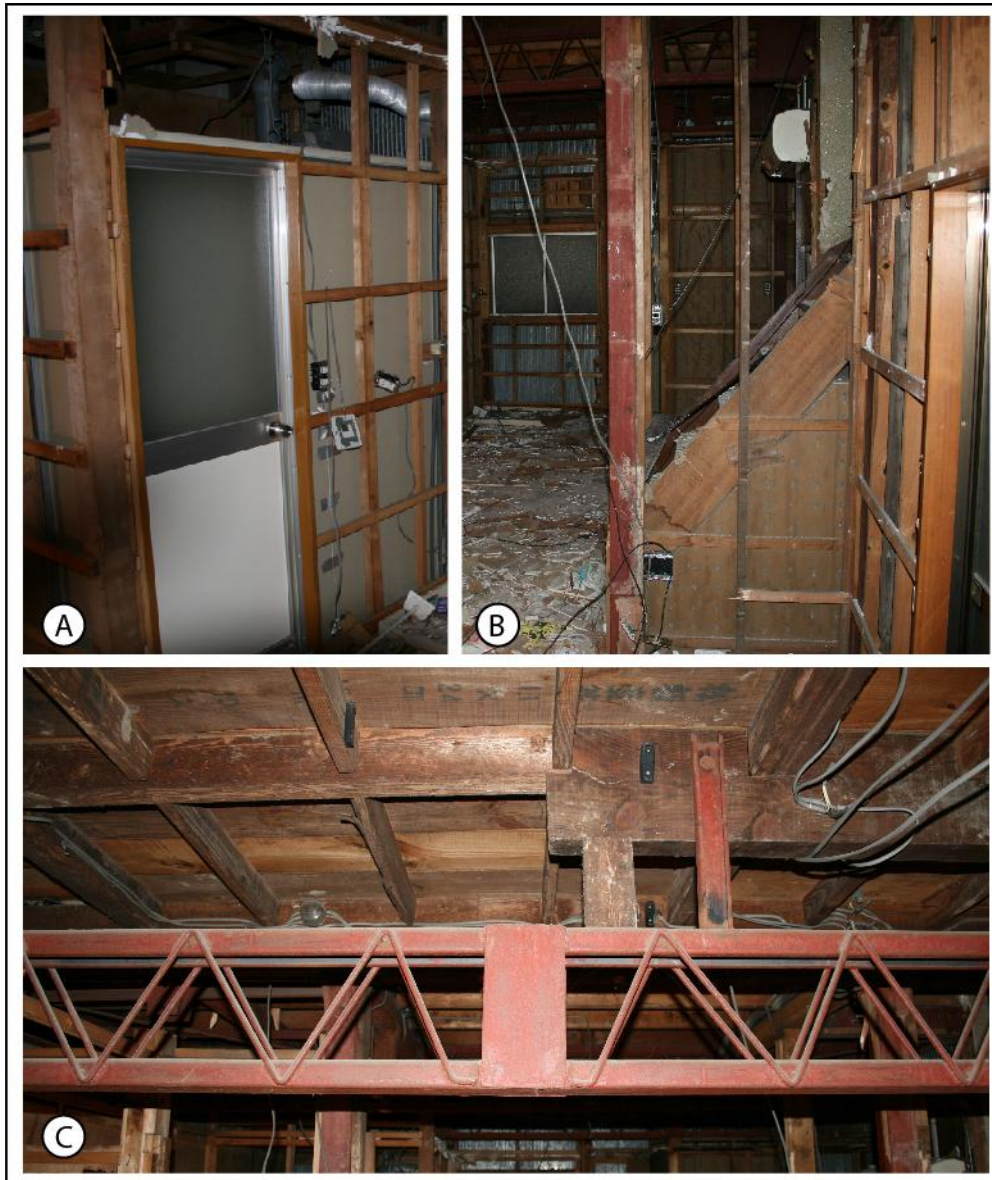
Fig. 8 Typical timber-frame structure house, which has been reinforced by a metallic structure during the Showa period (1926-1989). We can also appreciate the external wall panels made of painted steel. (Photos: C. Gomez, 2006)
