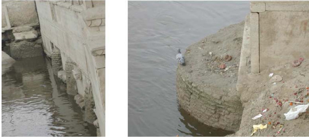
Figure 3: Masonry wells as foundation piles in Vrindavan
