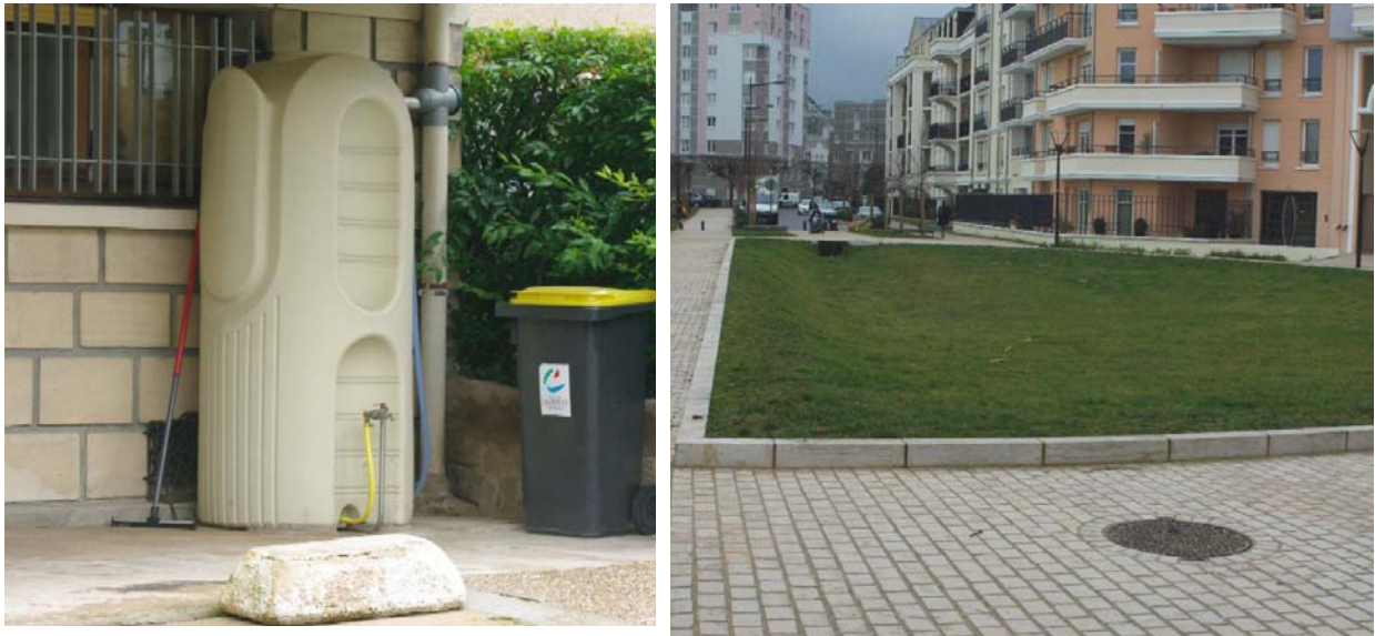
Figure 1 – Two examples of BMPs in France: a rainwater harvesting tank at the parcel scale in Champigny (Val-de-Marne), and an infiltration/overflow basin for a block of houses in Noisy-Le-Grand (Seine-St-Denis)
