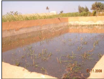
Photo 1: Planted drying bed at Cambérène (Abiola, 2009)
